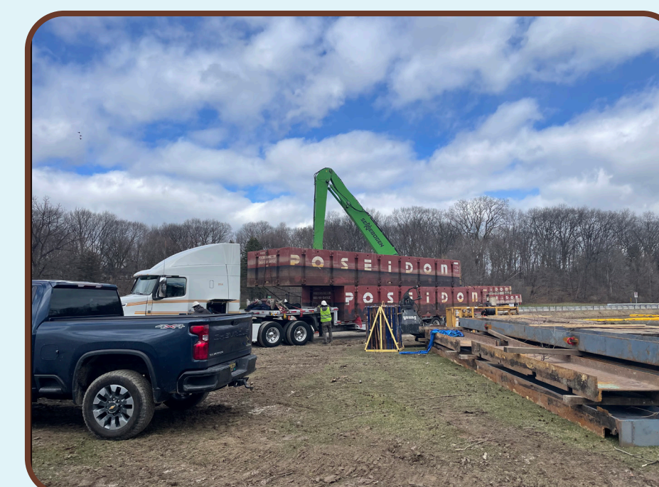
Delivery of barges at Wilcox Lake
