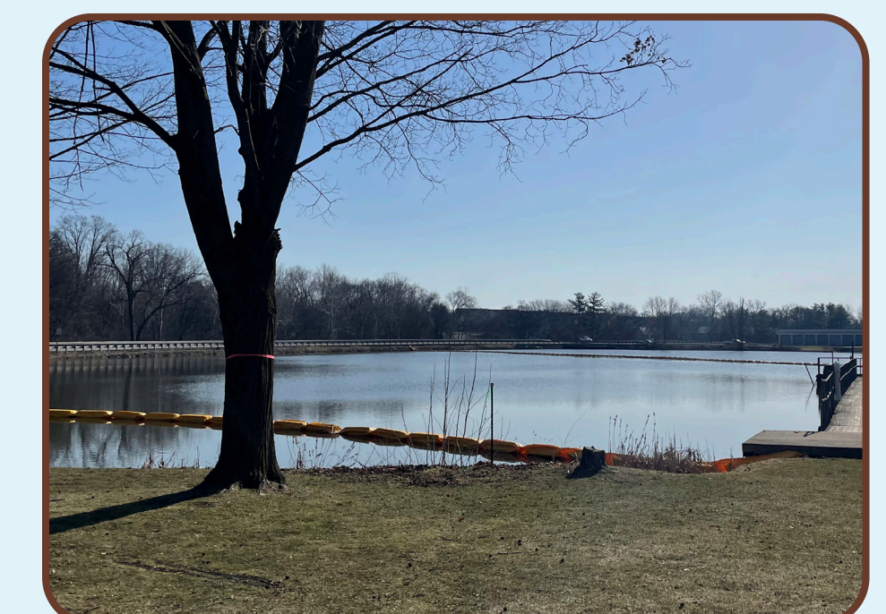
Turbidity controls in place at Wilcox Lake
