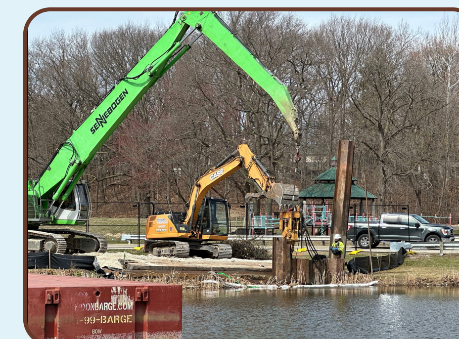
Installing transfer dock at Wilcox Lake
