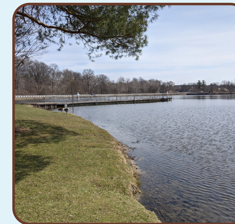
Existing conditions at Wilcox Lake
